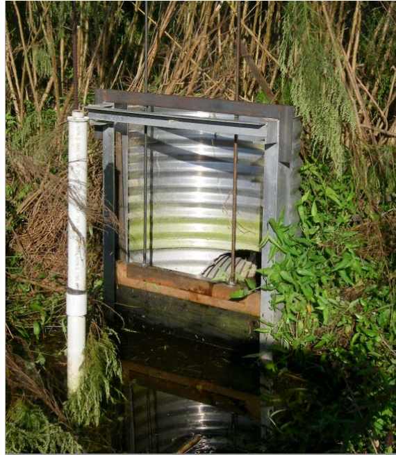
Figure 2. Wetland water retention BMP (flashboard riser) at wetland 4.
